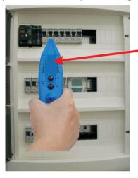
The Bar-Graph shows that the first circuit breaker of the first row has no signal on it. It buzz very slow too. The battery voltage is ok. You can go left and right and change row as you want to.
