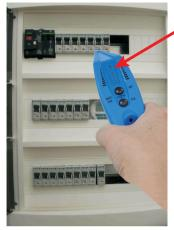
The Bar-Graph shows that the last circuit breaker of the first row has the signal on it. It buzz faster too. The battery voltage is ok.
